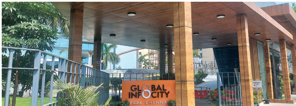
Improvements to the signage at GIPC, India, were conducted as part of asset enhancement initiatives at the business park.
