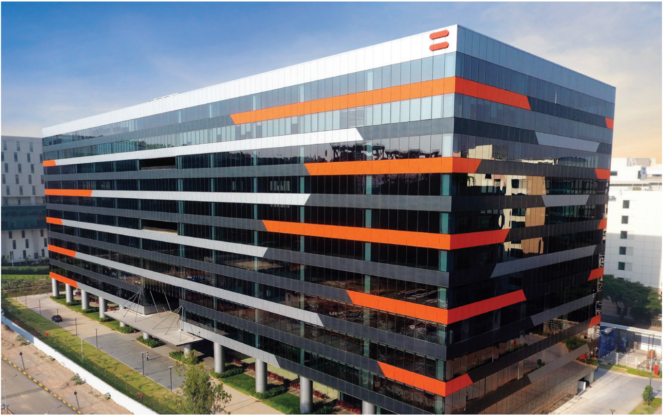
GTP, located in Bengaluru, is a Grade A business park which has achieved LEED Platinum certification.
