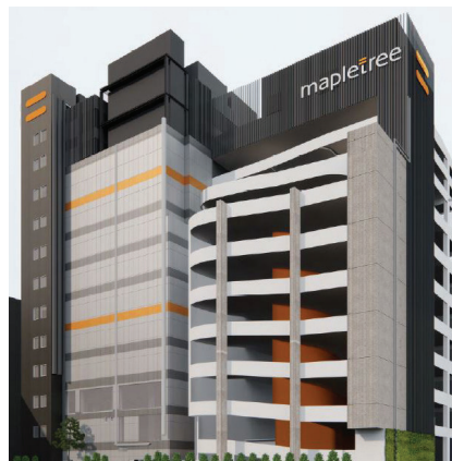
Mapletree's first data centre development in Fanling, Hong Kong SAR, will yield 20,140 sqm of GFA upon completion.
