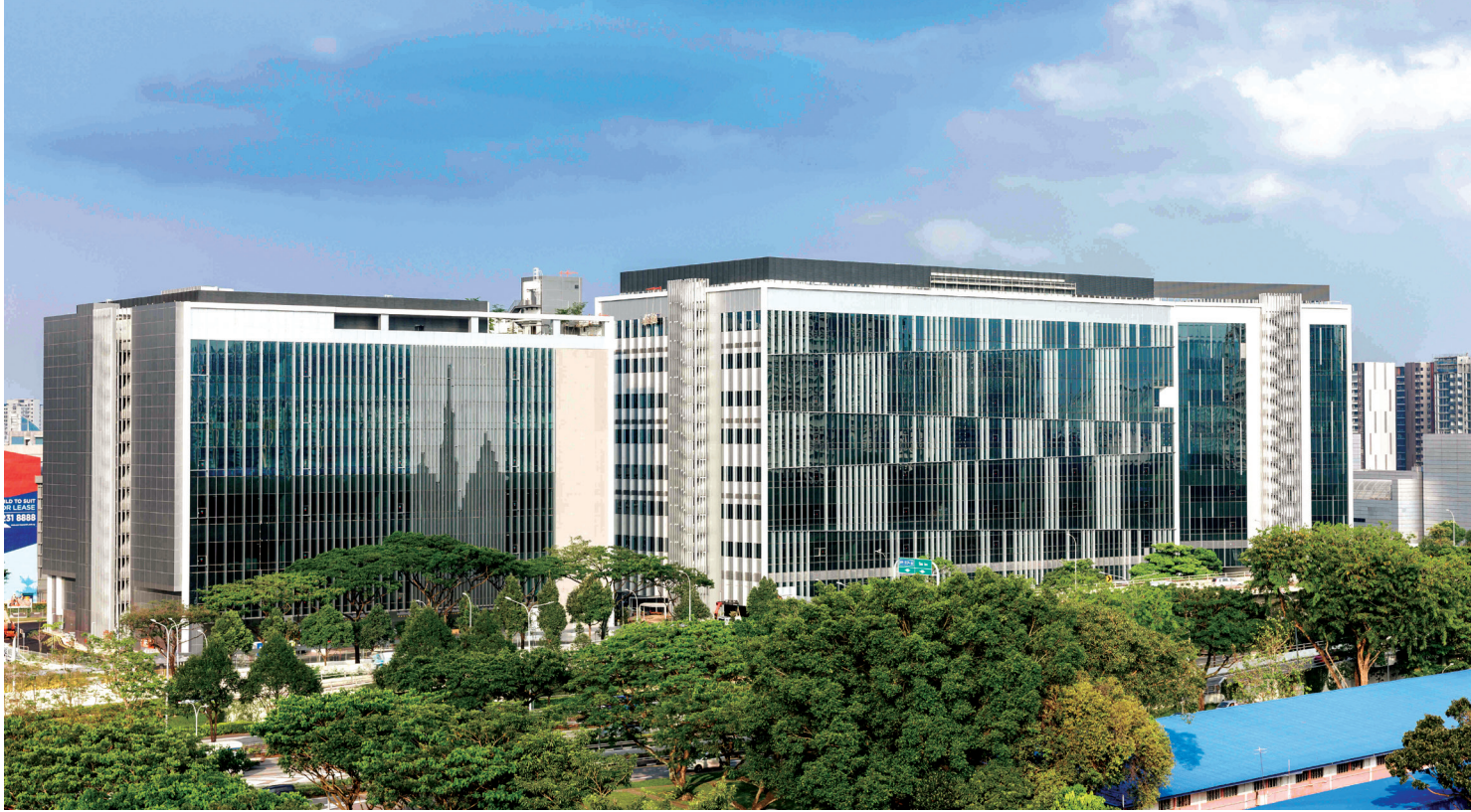
MIT completed its largest redevelopment project of flatted factories into a new high-tech industrial park, Mapletree Hi-Tech Park @ Kallang Way with an NLA of about 67,735 sqm.
